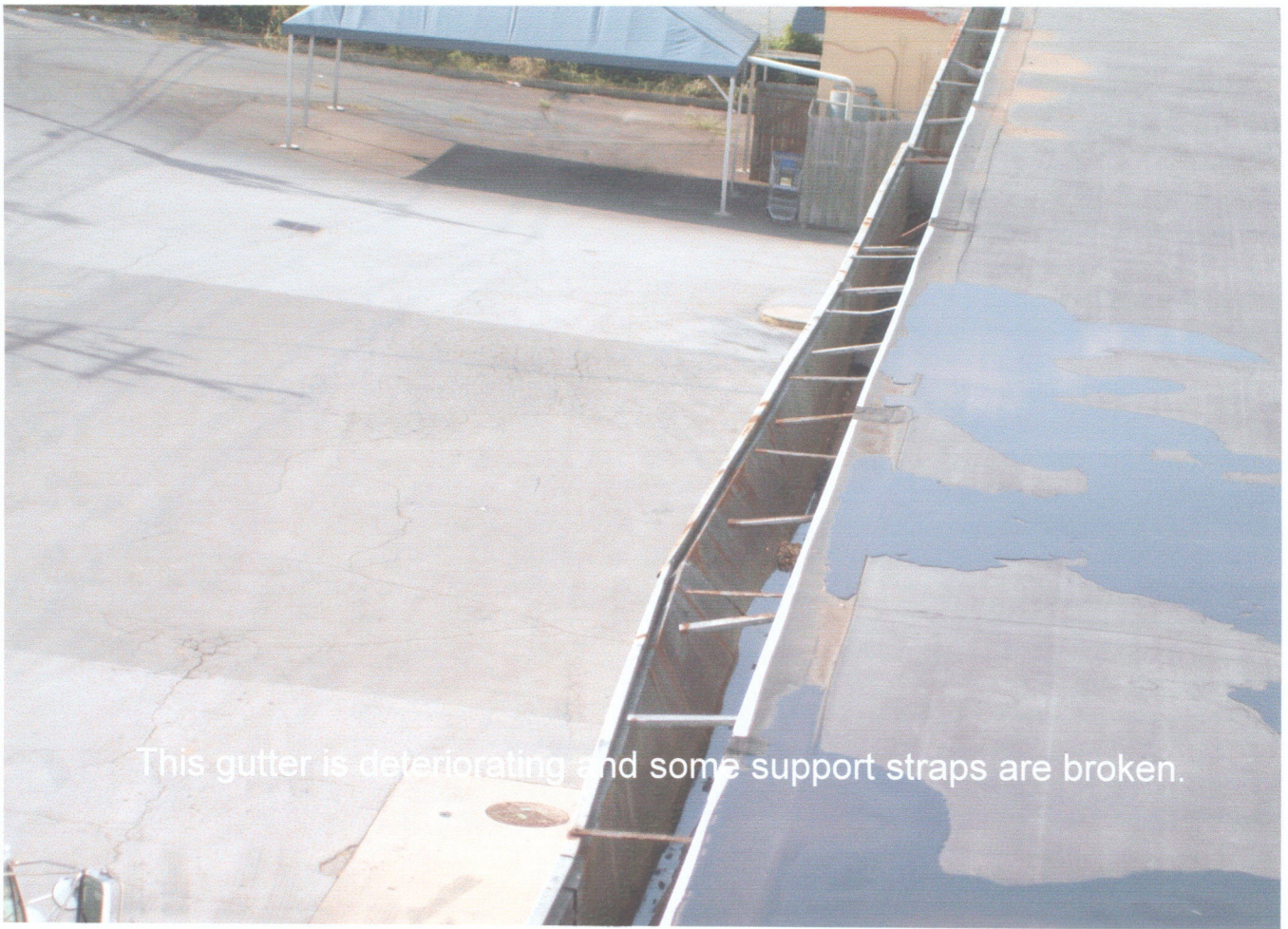
It appears that the EPDM roof was installed over the original roof.
