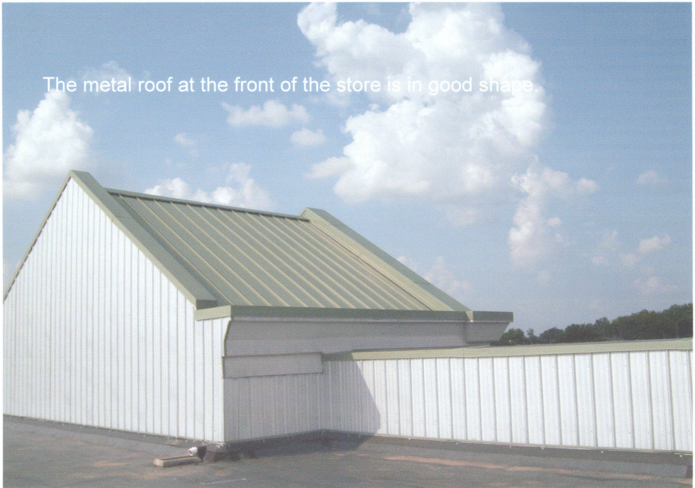
This roof is in fair to good condition.
